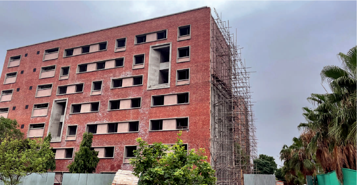
New hostel for women under construction
